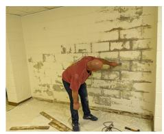
Sunday December 3, We attacked the bad walls. First, we laid plastic to collect the debris. Next, we began scraping. The the wall was cleaned with a wire wheel on a drill. To finish, we painted with a sealer.
