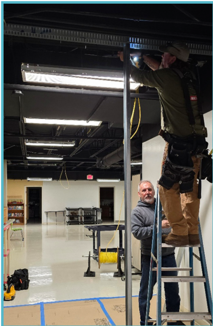
Discovery Zone Security Wall being Framed View is from Elevator into the Discovery Zone
